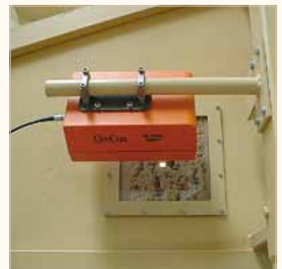
Side wall of dosing bin
